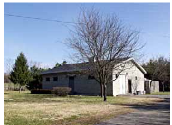
Existing South Elkhorn Pump Station
