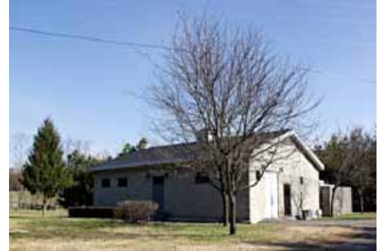
Existing South Elkhorn Pump Station
