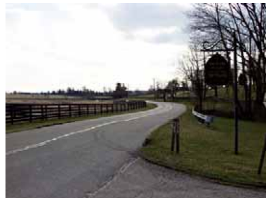
Delong Road/Richmond Road RSA
