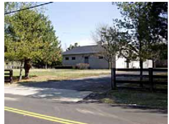
Existing South Elkhorn Pump Station
