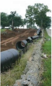
Above: Pieces of 42-inch pipe lay along a roadway for construction of a Kentucky American Water Co. water line from the Kentucky River in Owen County to Lexington.
