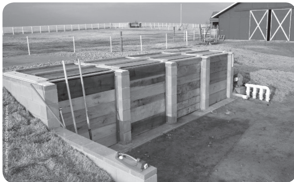
Aerated compost bays.
